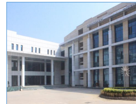
NCRB/CFPB new building At Mahipalpur, Delhi
